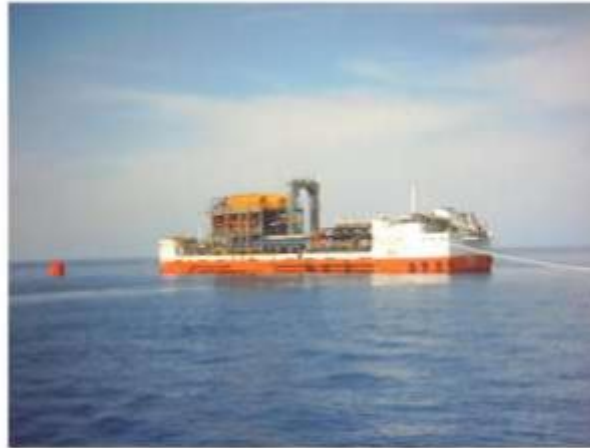
Figure 6.4: View of the Barge Mounted Desalination Plant.
