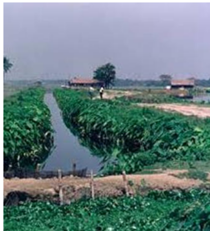
Fig:6.7 Sewage flow in pond through open channel
