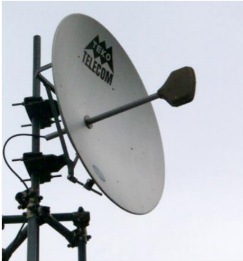
Figure 5.14: A solid dish antenna.
