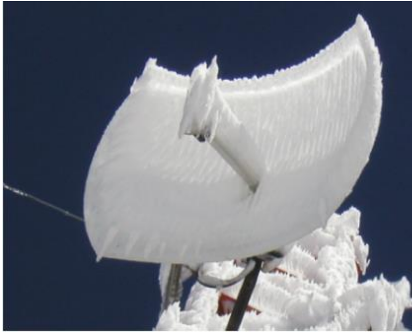
Figure 5.17: Effect of ice on a parabolic grid antenna
