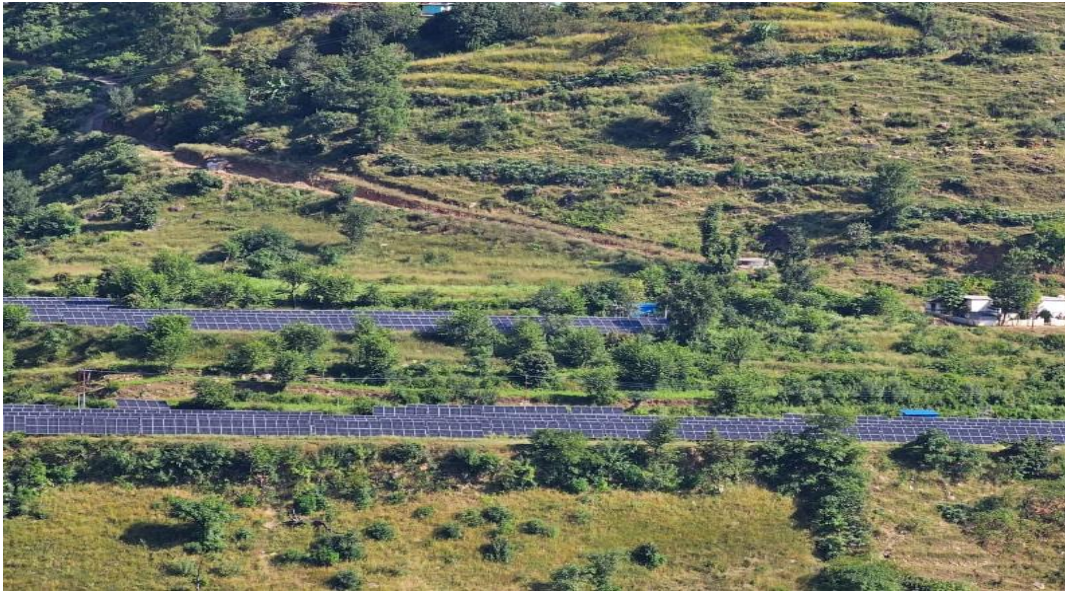
Fig 8.9: Solar Project by UREDA
