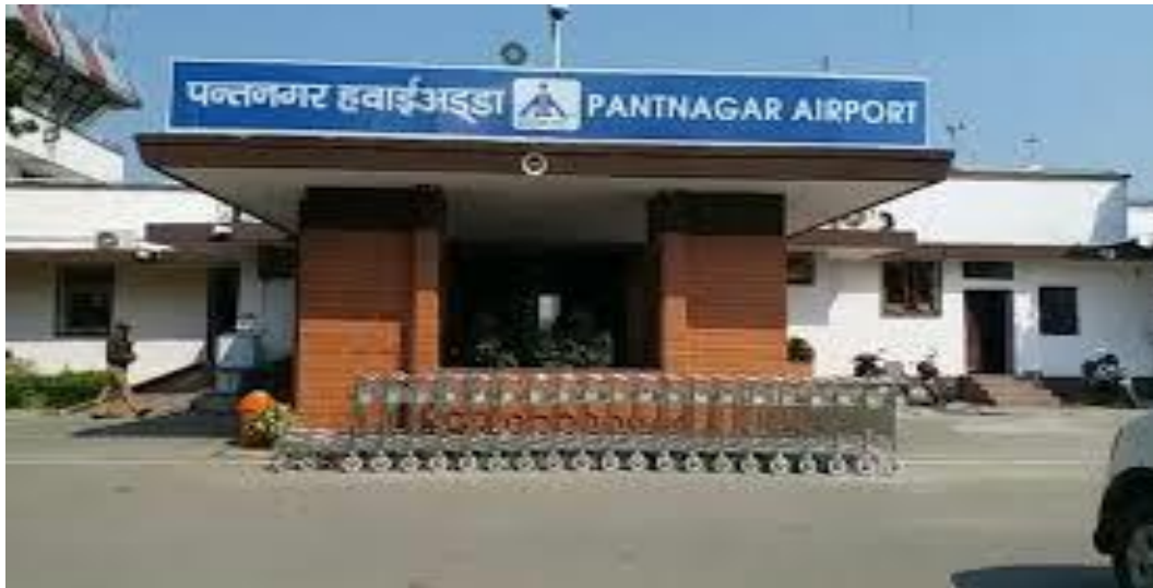
Fig 9.7 Pantnagar Airport (US Nagar)
