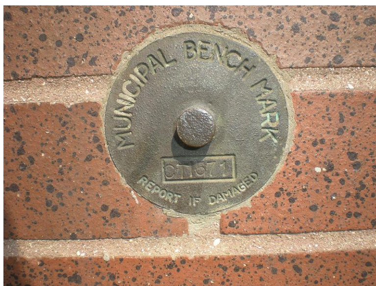
Fig. 4.5 City of Toronto benchmark disk in Canada.
