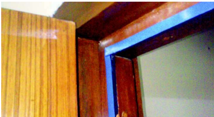
Figure 5.6 : A studio entrance door. Note how the door fits into the jamb against the blue gasket, making a soundproof seal. Photo courtesy: N.Ramakrishnan/Ideosync
