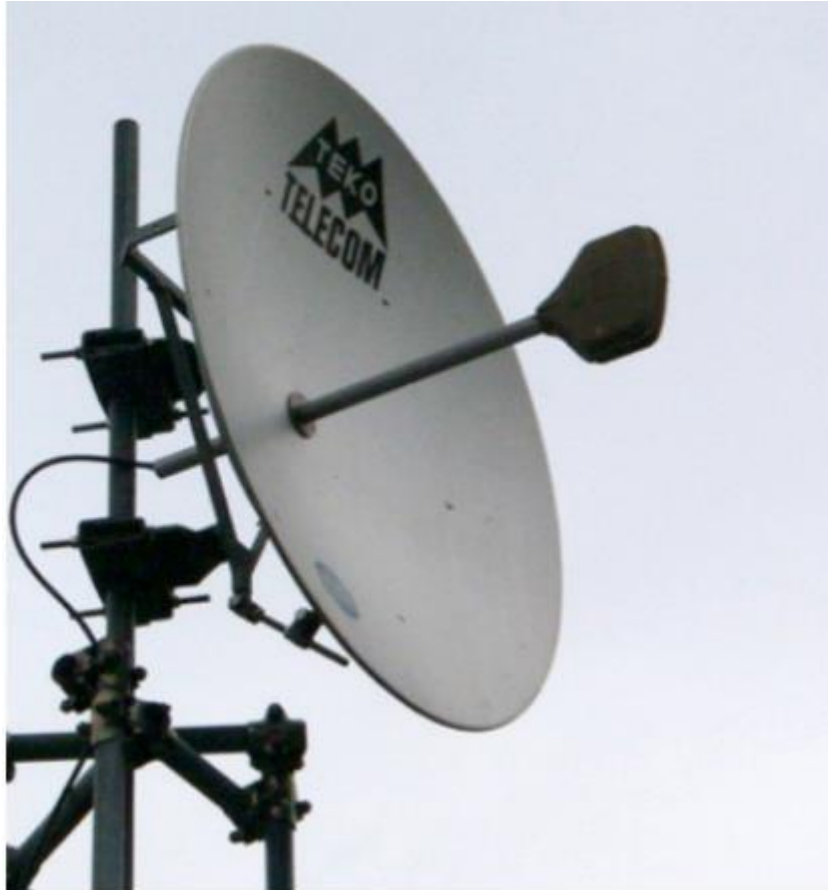
Figure 5.14: A solid dish antenna.
