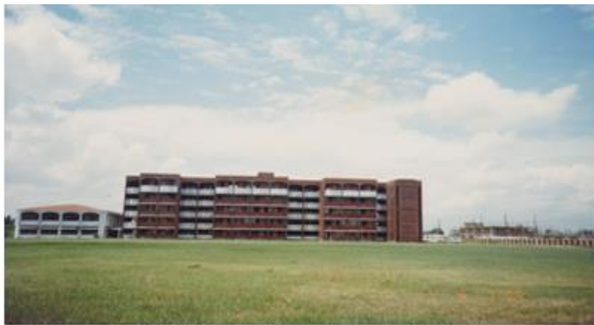
Figur:3- Physical Infrastructure under Construction.
